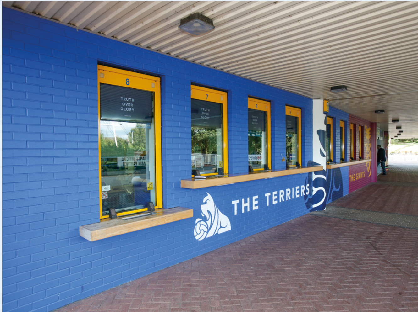
Figure 13 Ticket Office windows at the front of the Core Stand Lower Tier
