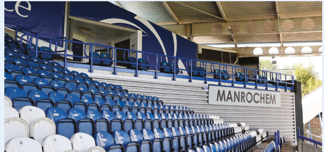
Figure 8 Raised platform for wheelchair users and their companions at the back of the Chadwick Lawrence Stand
